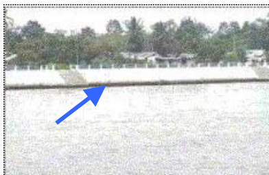
Figure 7 Retaining Wall to prevent abrasion
