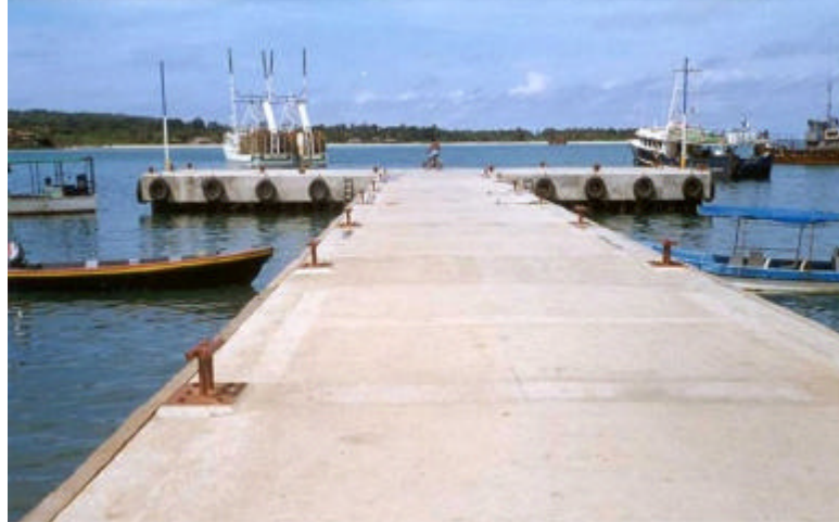
Wharf constructed by Danida Transport Programme in Corn Island
