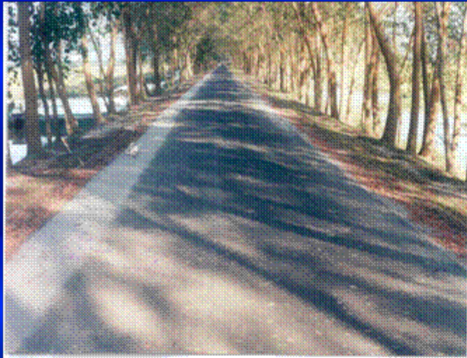
Improved Rural Roads
