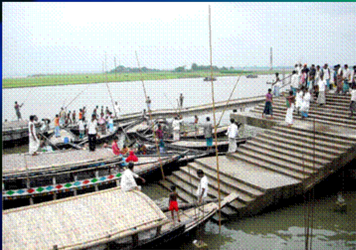
Constructed River Jetty
