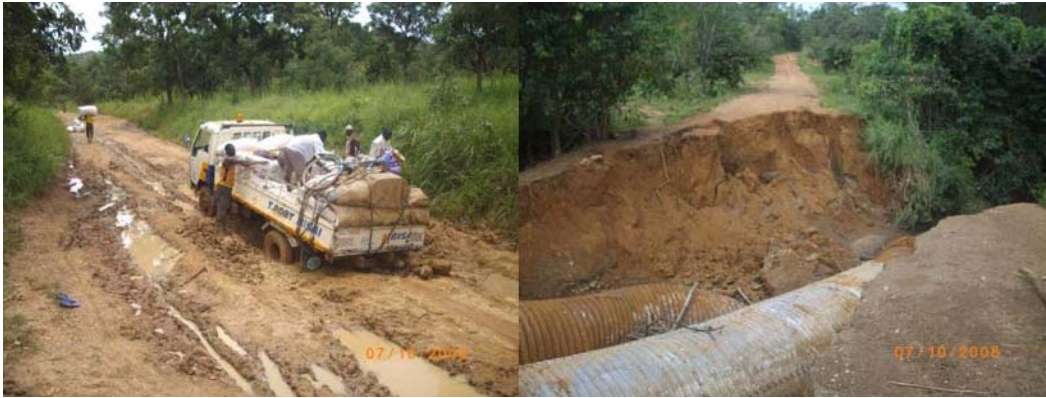
Picture: Transferring a cargo of maize because the vehicle got stuck (left), and the collapse of a bridge (right) Fofiri, Tignère (Adamawa), October 2008
